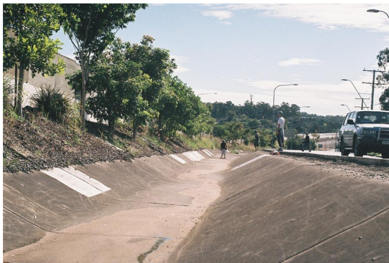
Figura 7.4.3. Cuneta en una carretera. Recuperado de: http://www.skateboardracing.org.au/forum/topics/ditches-in-the-sunshine-state
