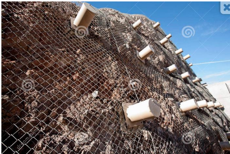
Figura 6.5.2. Patrón de anclaje de una anchored mesh . Recuperado de: http://www.dreamstime.com/royalty-free-stock-images-steel-mesh-anchor-rockfall-protection-image29441419
