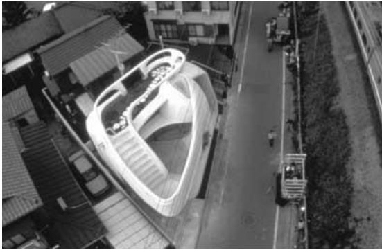
4.10 Truss Wall House Machida-city, Tokyo, Japon, 1993
