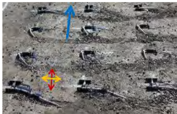
SENSORES ASG (Asphalt Strain Gages)
