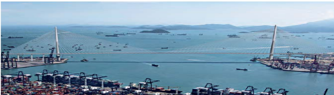
Figura 9: Puente Stonecutters, Hong Kong
