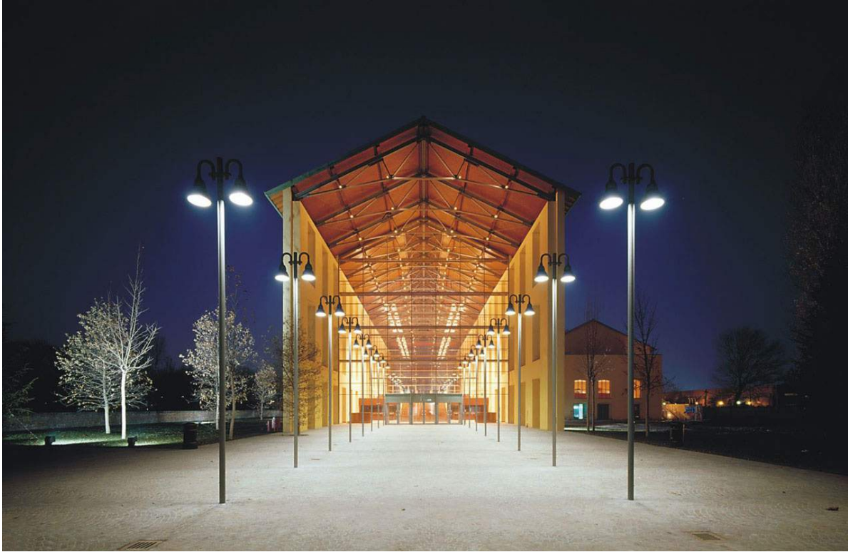
Fachada principal Auditorium
