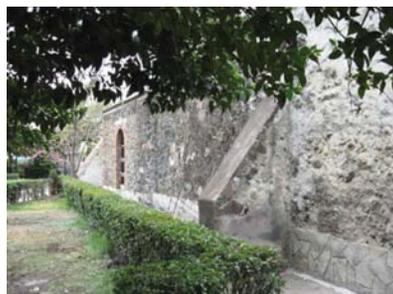
MURO Y CONTRAFUERTE EN PIEDRA BRASA CON RAJUELEADO Y LAJAS. CONTRAFUERTE CON APLANADOS EN CEMENTO ARENA EN LA PARTE SUPERIOR. RODAPIÉ EN CEMENTO-ARENA CON ENTRECALLE IRREGULARES.
