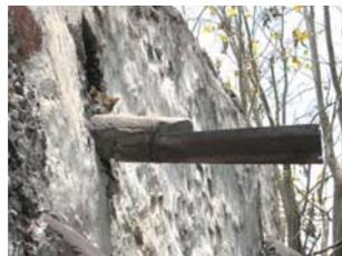
GÁRGOLA IMPROVISADA CON PIEZA DE LÁMINA Y BASE DE CONCRETO.
