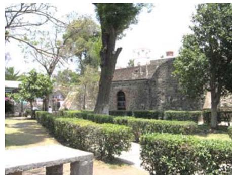
FACHADA SUR CON MUROS Y CONTRAFUERTE EN PIEDRA BRASA CON RAJUELEADO. GÁRGOLA IMPROVISADA A BASE DE LÁMINA ACANALADA.
