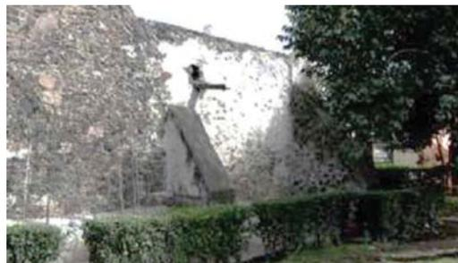
MURO Y CONTRAFUERTE EN PIEDRA BRASA CON RAJUELEADO Y LAJAS A DISTINTAS ALTURAS. GÁRGOLA IMPROVISADA A BASE DE LÁMINA ACANALADA.
