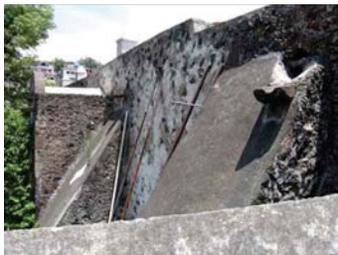
FACHADA ALTAR LATERAL NORTE Y CONTRAFUERTE EN PIEDRA BRASA y RECUBRIMIENTO APLANADOS EN CEMENTO-ARENA. ALTAR LATERAL Y MURO DE PIEDRA INTERCUPULAR CON DESPLOME.
