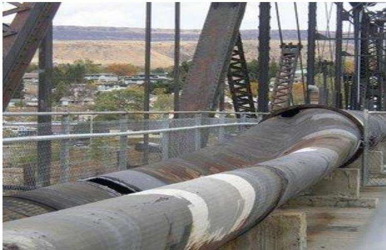
FIGURA 3. 1 TUBERÍA DE ACERO HELICOIDAL CON FALLA POR APLASTAMIENTO
