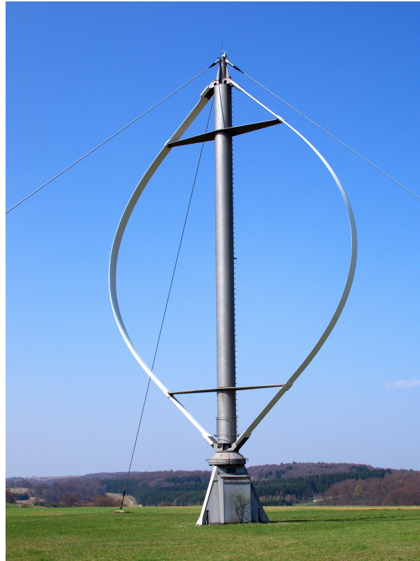
Figure 1.2: Darrieus rotor of two blades
