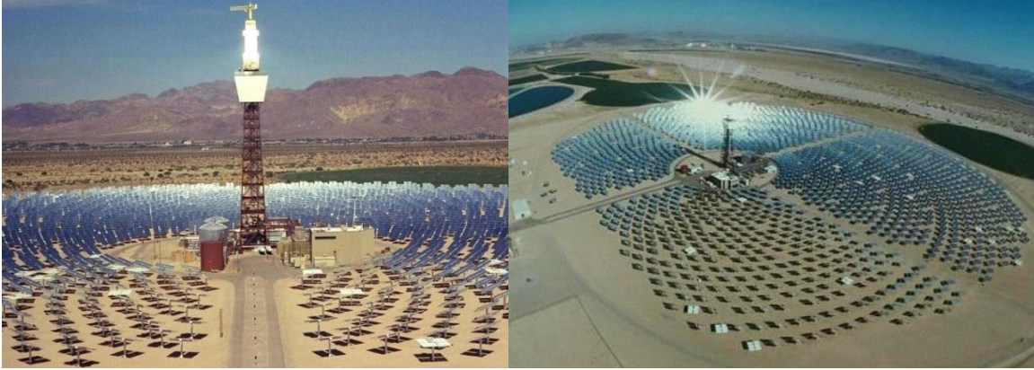
Figura 1.14: Planta Solar One, Barstow CA.
