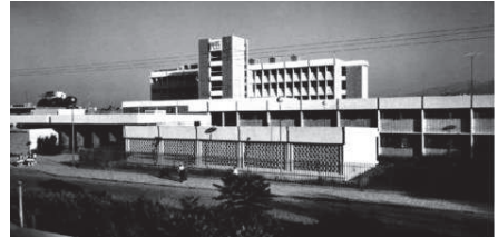
HOSPITAL DE GINECO-OBSTETRICIA EN S.L.P
