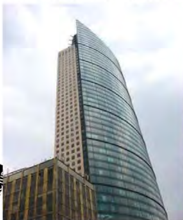
VISTA 1: TORRE MAYOR
