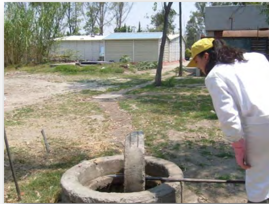
Figura. 3.15. Recorrido del colector principal
