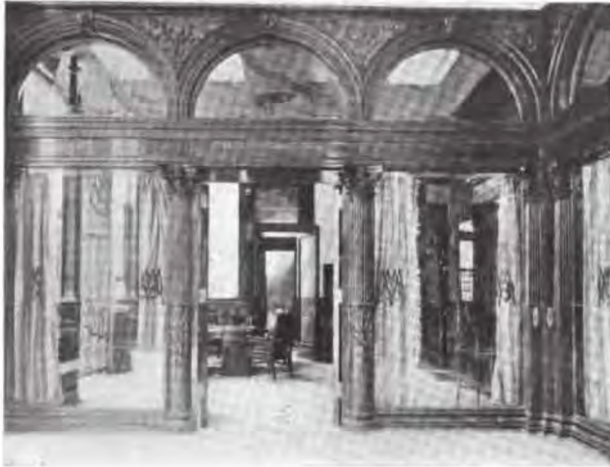
Entrance to Manager's Office.
