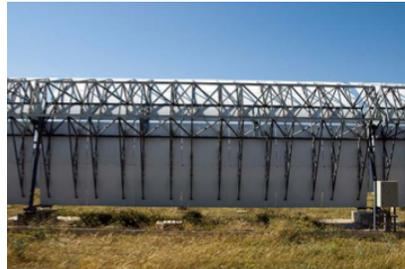
**Figura 2.4** Estructura Torque-Box del colector EuroTrough ET-100 y ET-150
