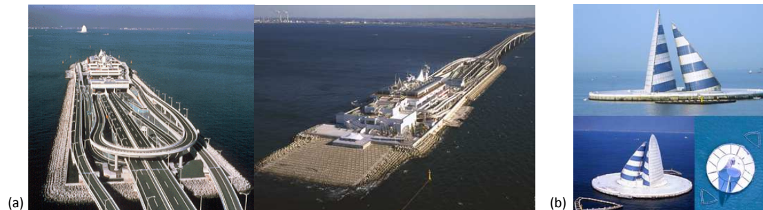
Figure 2.17 Artificial islands in the Tokyo Bay Aquiline: (a) The Kisarazu Island joins the subsea tunnel and the bridge; (b) The Kawasaki artificial Island works as ventilation towers. (dvice.com & findery.com)
