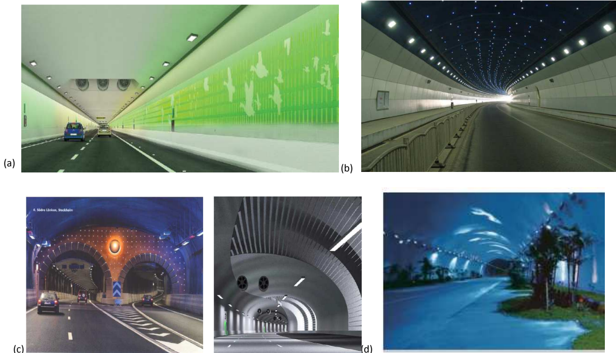
Figure 4.51 Visual designs in road tunnel: (a) Fehmarnbelt Tunnel, Denmark-Germany; (b) Dongshan Tunnel, China; (c) Södra Länken Tunnel and Stockholm bypass, Sweden; (d) Qinling Zhongnan tunnel, China
