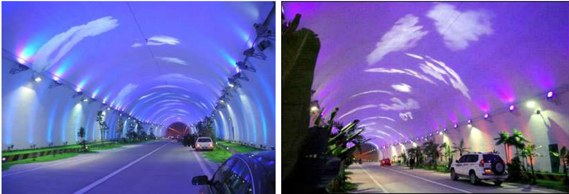
Figure 2.10 Interior design of the Zhongnanshan Tunnel (China.org.cn)
