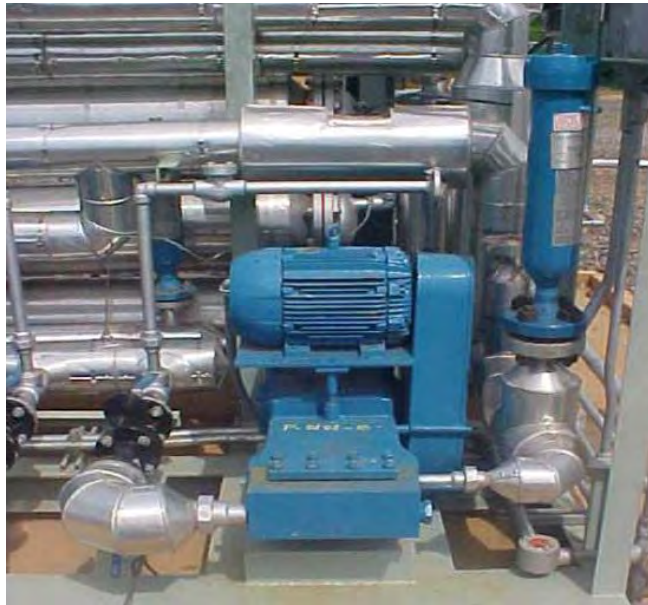
Fig.51.- Bombas de glicol pobre. Fuente.- Copyright 2007, NCT, Energy Group. All rights reserved.
