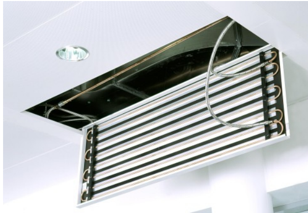
Figure 1.5: Radiant panel mounted inside a false ceiling (opened to show the inside).
