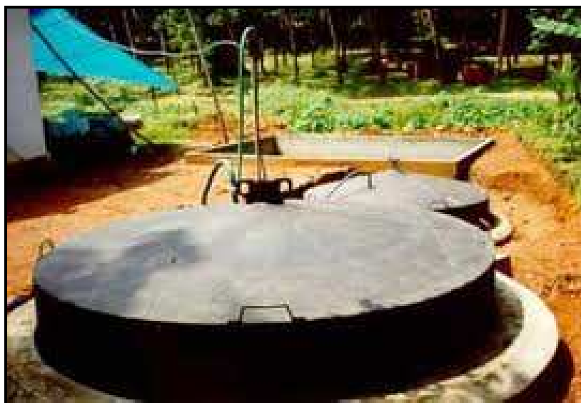
Figura 2.20 Reactor vertical tipo indio (PAKS, 2011)
