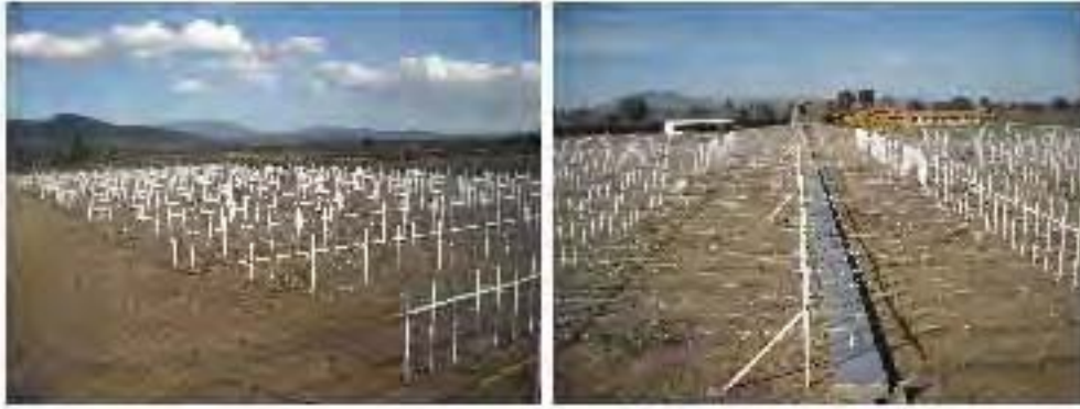
Figure 4.1: Pictures of the MEXART facilities. ( Left ) The antenna, showing the ensemble of the 4096 dipoles. ( Right ) facilities at the site: antenna, control room, laboratories, staff offices and guest house for students and visitors.
