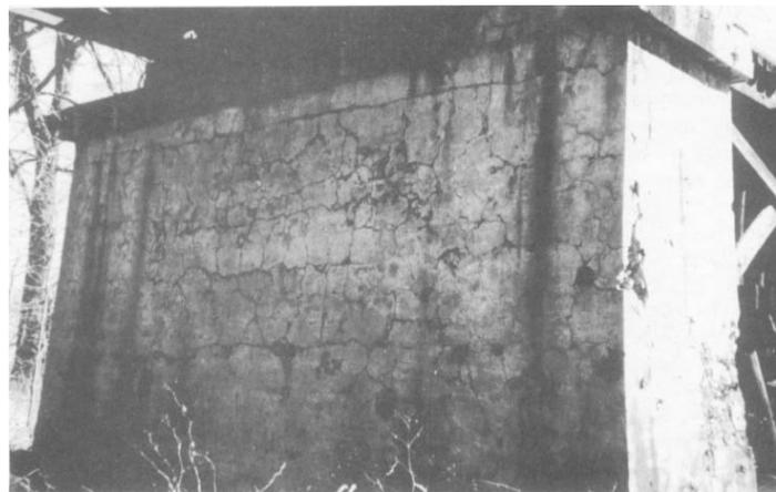
*Fig. 2.14 Agrietamiento en la subestructura (Departments of the Army and Air Force of United States, 1994)*
