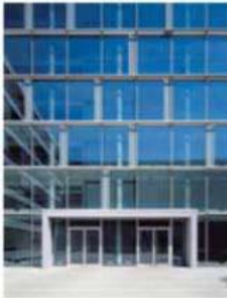
Frankfurt Police Headquarters, Germany Architects : KSP Engel and Zimmerman
