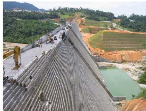
pre-cast block forms for 0.6m d/s steps for SLM in 3m lifts
