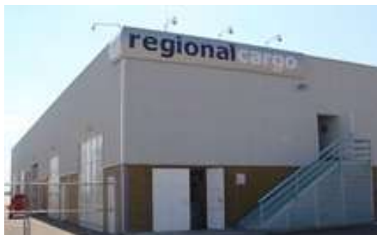
Figura 4.28 Terminal carga Regional Cargo QRO
