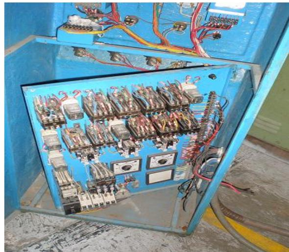
Figura 4.2.1.2 Interior tablero de control
