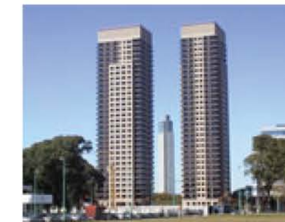
Torres River View
