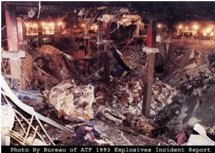
Photo By Bureau of ATF 1993 Explosives Incident Report
