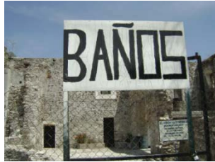
Vista Fachada principal
