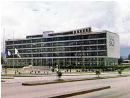
Foto No. 21: Palacio Municipal, Guatemala (1958)
