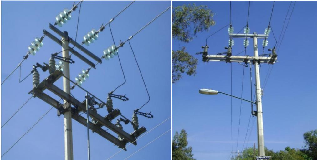
**Figura 1.23 Cuchillas tripolar ALDUTI.**
