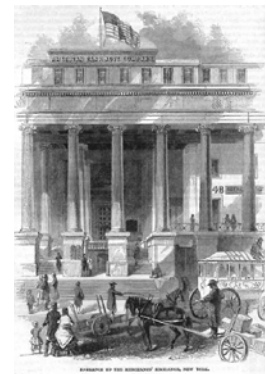
Fachada principal American Bank Note Company
