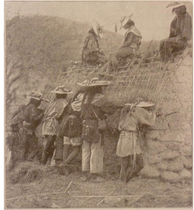
Praying while Putting a New Roof on a God-house in Ratontita.
