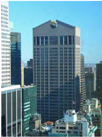
Sony Building Philip Johnson 1982
