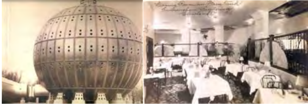
Fig. 5. Fachada e interior del “Steel Ball Hospital” 3
