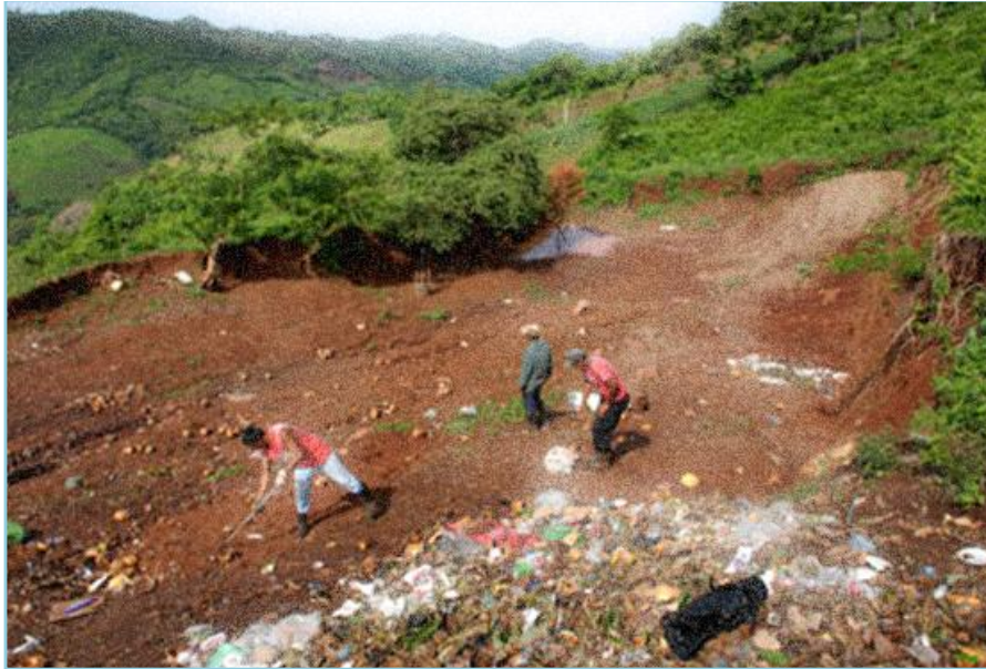
Figura 1.16 Relleno manual
