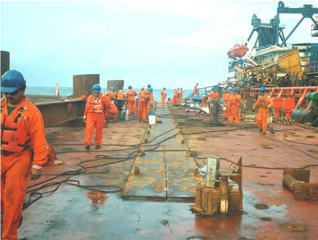
FOTOGRAFÍA 4.33 PLACA Y GUÍAS DE DESLIZAMIENTO PARA ARRASTRE Y DESEMBARQUE EN PATIOS DE TUXPAN, VER.
