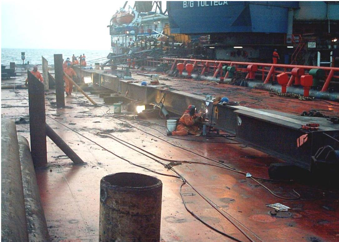
FOTOGRAFÍA 4.26 VIGAS DEL EJE A DEL MARCO SOPORTE
