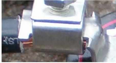
FIGURA 4.7 AREA DE COBRE A PROTEGER EN EL ELECTRODO.
