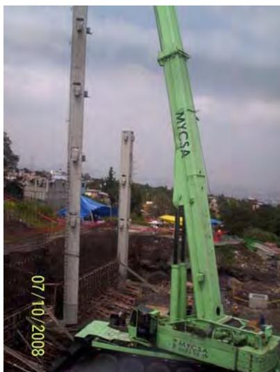
*FIGURA 20. MONTAJE DE COLUMNA CON GRÚA*
