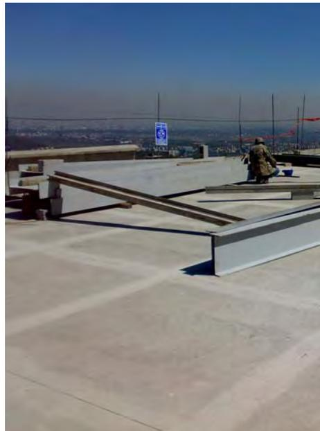
*FIGURA 34. LOSAS,  $F'c = 350 \text{ KG/CM}^2$*
