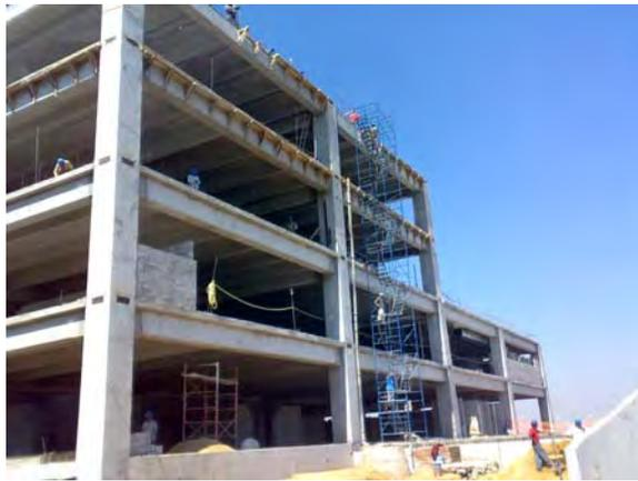
*FIGURA 35. SISTEMA DE LOSAS Y COLUMNAS*
