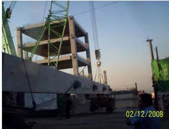
*FIGURA 32. IZAJE DE COLUMNAS*
