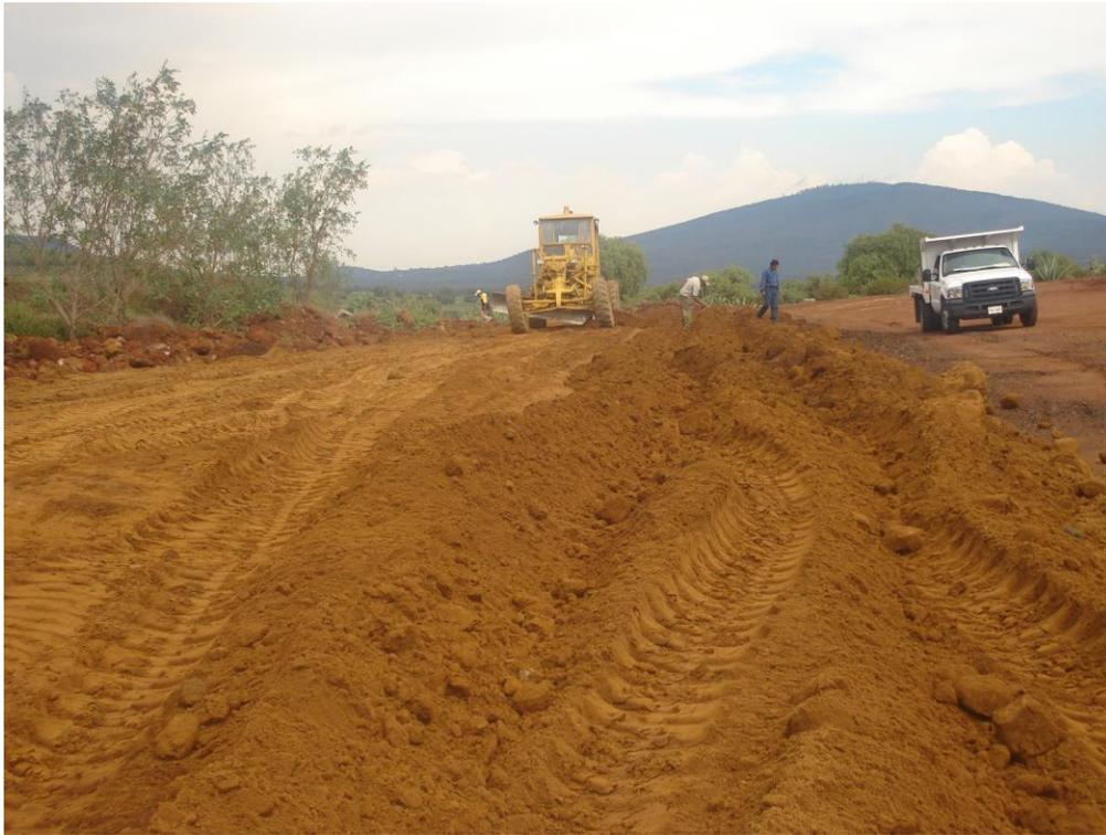
FIG. 2.1.1.2 TENDIDO DE MATERIAL (TEPETATE)
