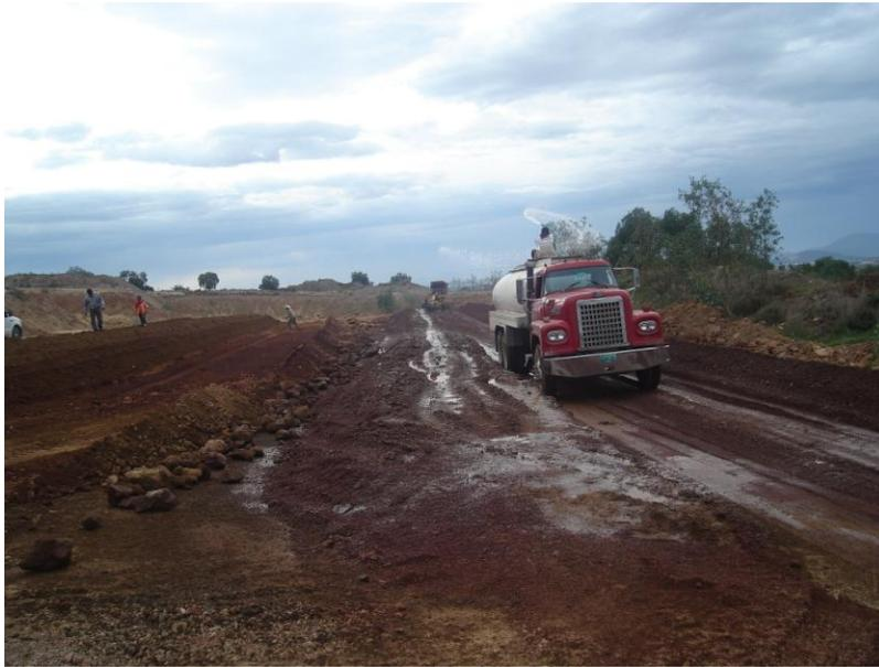
FIG. 5.2.1.1 INCORPORACION DE HUMEDAD A MATERIAL PARA CONFORMAR BASE
