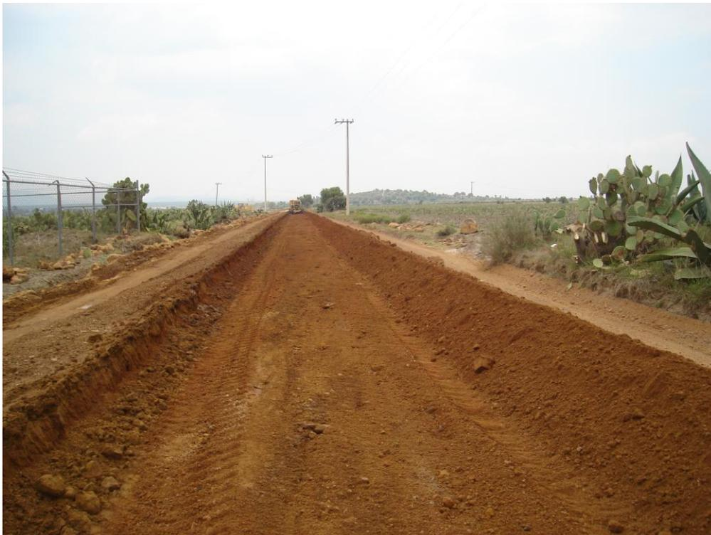
FIG. 5.9.1 CONFORMADO POR MEDIOS MECANICOS DE BASE GRANULAR CASCAJO-TEPETATE EN PROPORCION 70-30
