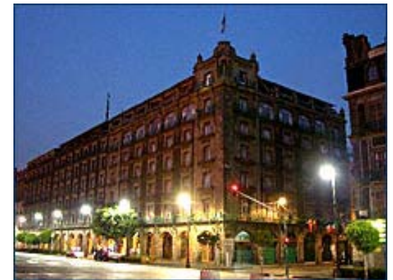
F-21 Hotel Best Western Majestic Centro Histórico, vista exterior, Fachada principal
