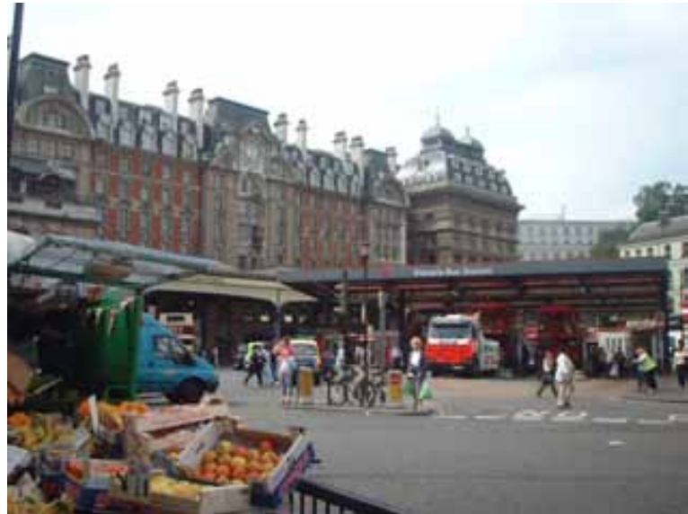
Fig.3 Central de autobuses Victoria Bus Station, Londres.
