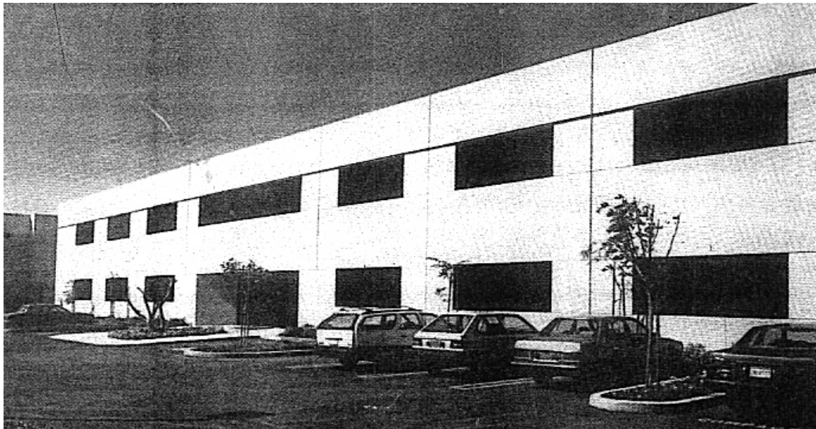
Figura 1.7 Nave Industrial General Electric. Pasteie. México.
