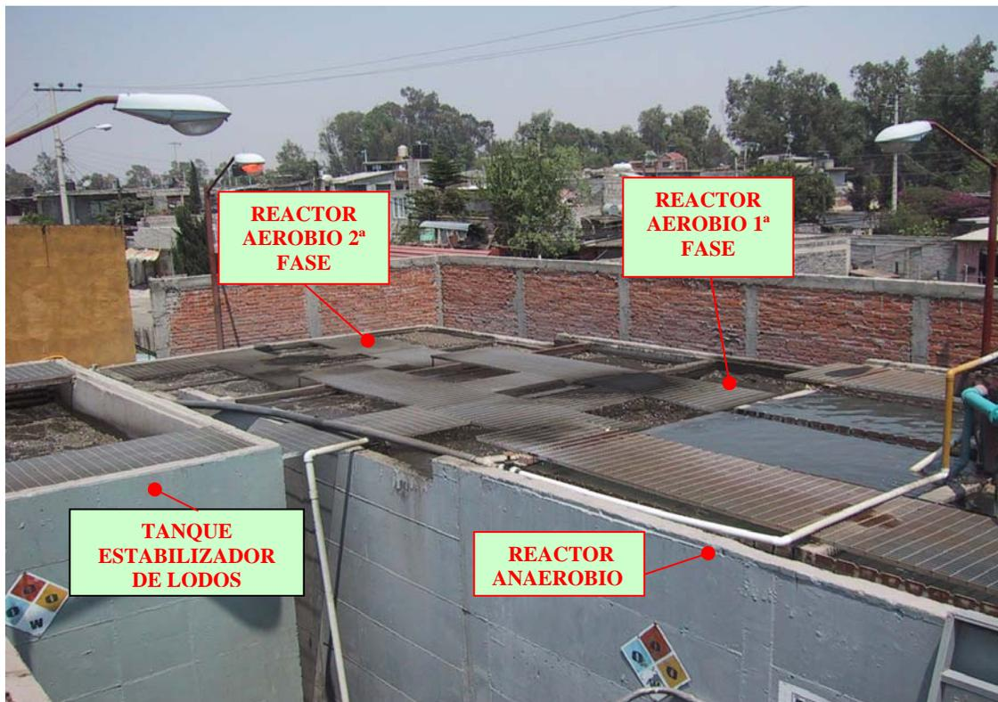
*Figura 2.13 Reactor aerobio*
