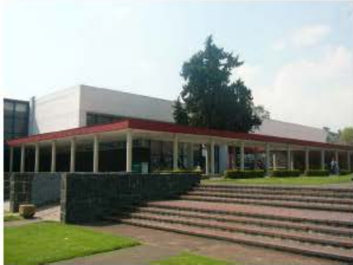
: Vista fachada principal
