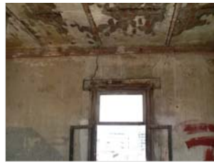
F-39 VISTA INTERIOR VENTANA 14-01-05
