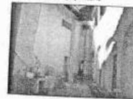
(F9) PATIO INTERIOR
