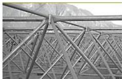
Fig. 34- Losa reticular tridimensional.
