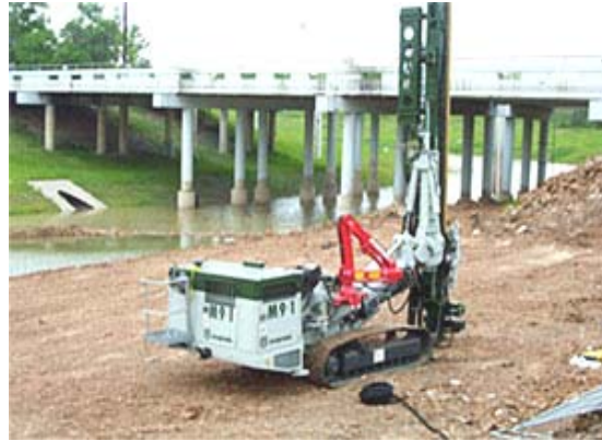
Fig. 1.15 Empleo de Jet Grouting.
