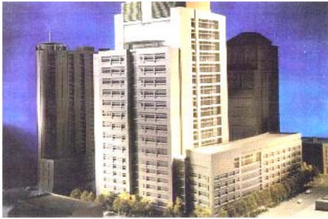
Fig. I.8-2. Vista del "Seattle building"
