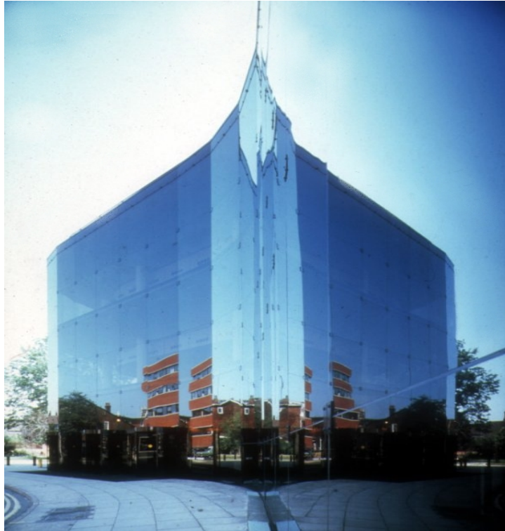
Fig. 17 Fachada del Willis Faber and Dumas Headquarters
