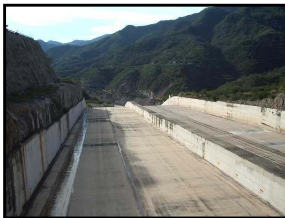
Fig.III.71.-Canal de Descarga Aguamilpa, Nayarit
